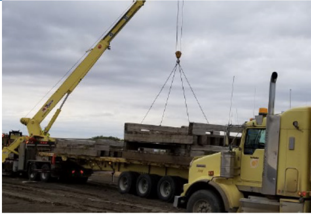
Offloading bridge - Km 255+680– Sept 20, 2018
