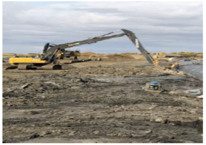
Backfill crew cleaning up geo tech – Sept 20, 2018
