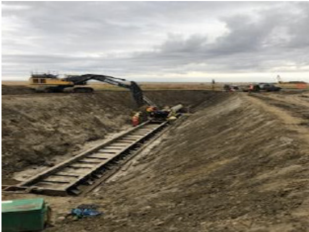
Track bore crew working beneath train tracks – km 175+200 – Sept 20, 2018
