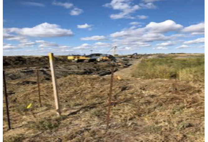
Crew prepping for tie in – SF 97 –Sept 19, 2018
