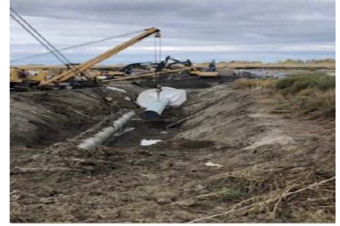
Welding tie - in – SF 97 – Sept 20, 2018
