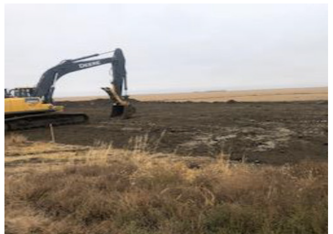
Topsoil being stripped – SF 158 – Sept 21, 2018
