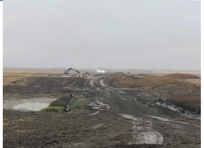
Excavators loading rock trucks – km 164+400 – Sept 21, 2018
