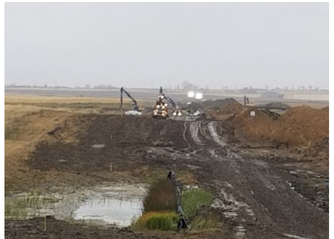
Working on aquadam – km 164+500 – Sept 21, 2018
