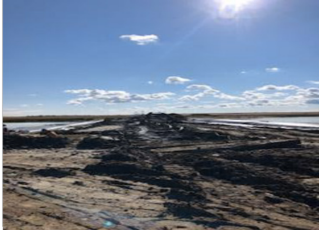
Backfill at aquadam – SF 97 – Sept 19, 2018
